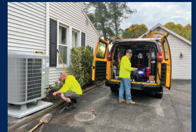
Dean Faiola and Adam Lambert installing a new unit
