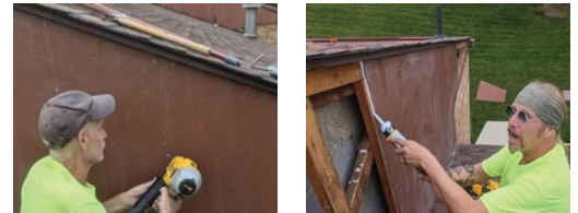
Jason Hare and Greg Moyer repair and re-side the buildings
