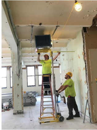
CF Acri employees Kenny Myers (on ladder) and Dylan Gilbert (operating the duct jack) work on the Menaker Building project.
